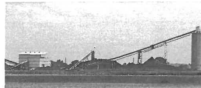
Knight Hawk Coal Mining Perry County, Illinois 3,000MW solar plus battery storage project being developed on surface coal mines in southern Illinois.
