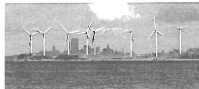
Steel Winds Lackawanna, New York 20MW wind project sited on former Bethlehem Steel factory.
